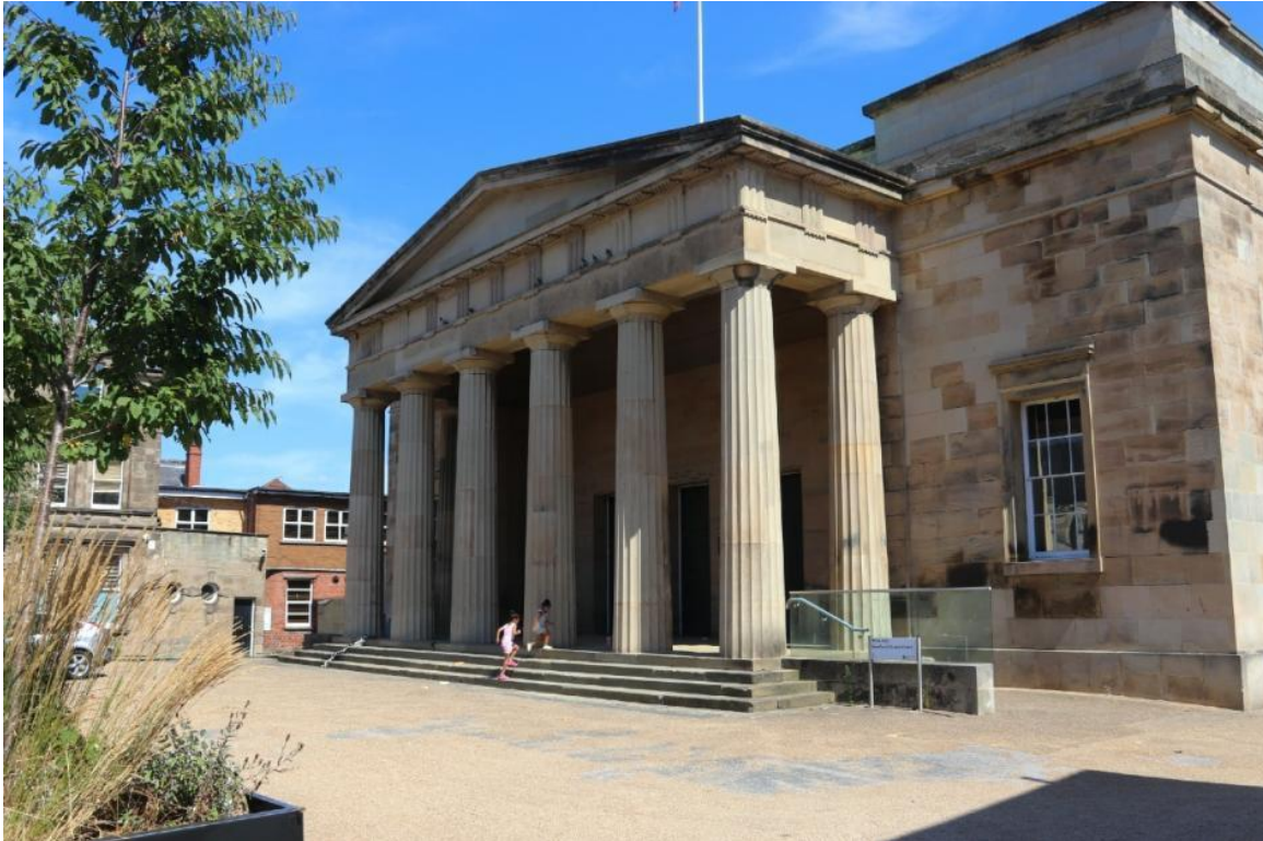
Fig 11: Front of Shirehall building
